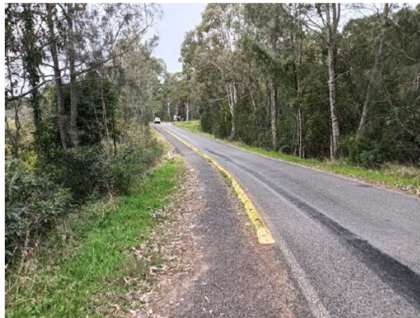
Figure 15 – View of central section of Mustons Road (narrow section)
