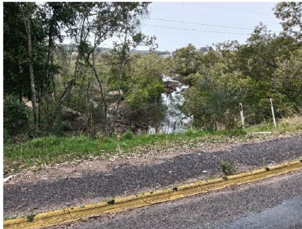
Figure 14 – View from Mustons Road of vegetation to the east (at culverts)
