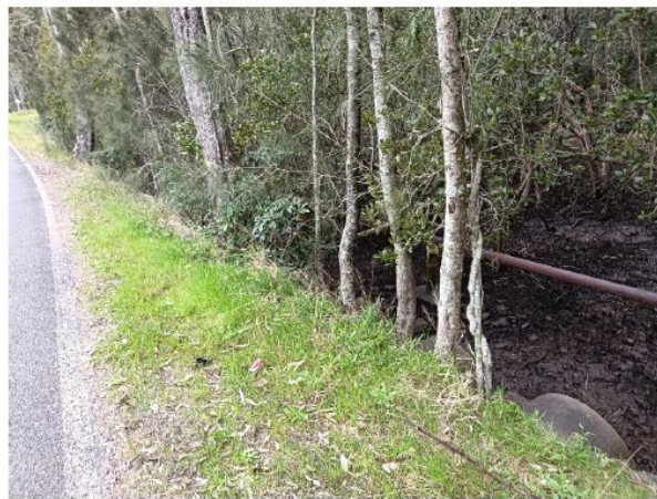
Figure 12 – View from Mustons Road of vegetation to the west (at culverts)
