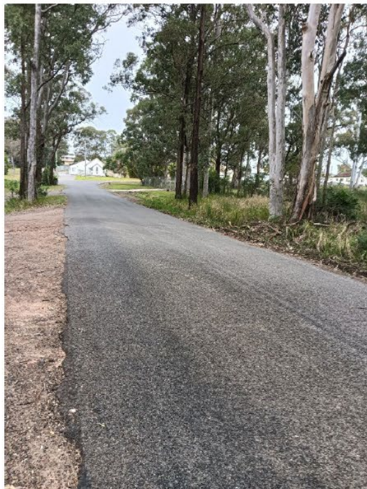
Figure 7 – View of northern section of Mustons Road
