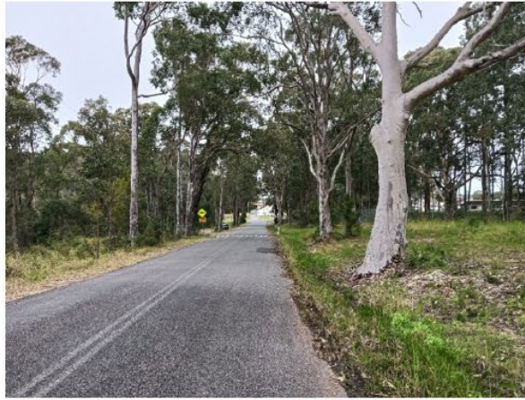
Figure 3 – View of southern section of Mustons Road
