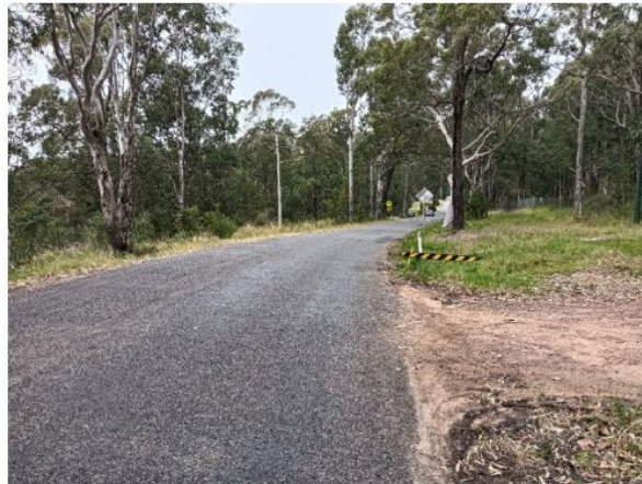
Figure 4 – View of southern section of Mustons Road
