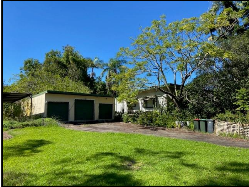
Image 1: Existing structures on the site proposed for removal
