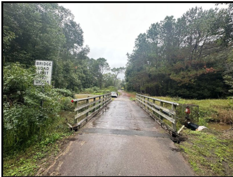
Photograph 3: Bridge crossing over Grahamstown Drain
