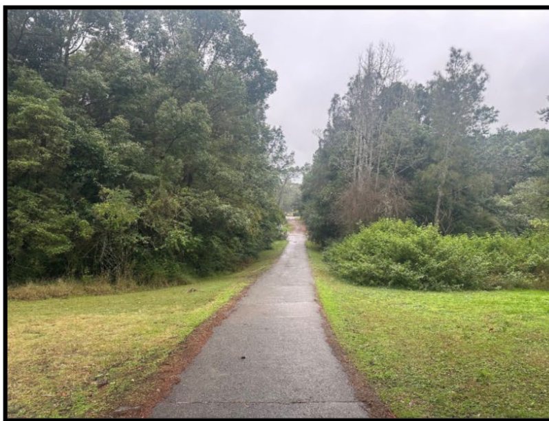
Photograph 2: Right of carriageway as viewed from 60m along road
