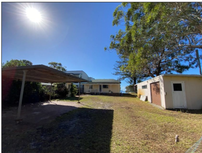
Photograph 2. Existing dwelling and ancillary structures looking east
