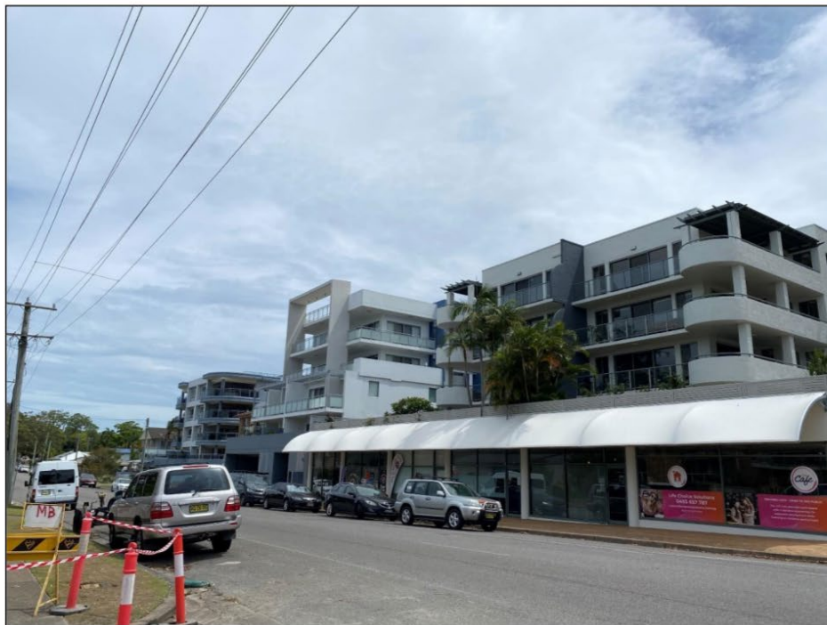
Figure 4. Existing shop top housing directly adjacent to the site across Soldiers Point Road
