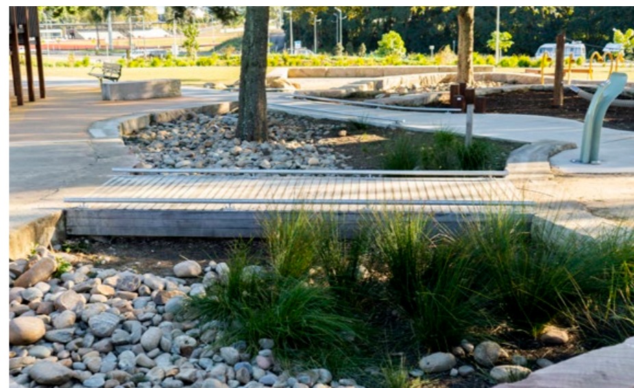
Rain gardens and crossings (Harold Gregson Park / Moir Studio)
