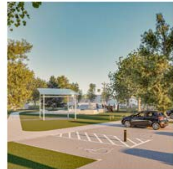
Accessible parking off Ferodale Road
