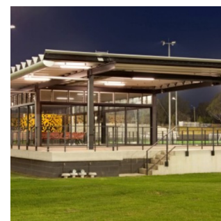
Communal covered space
