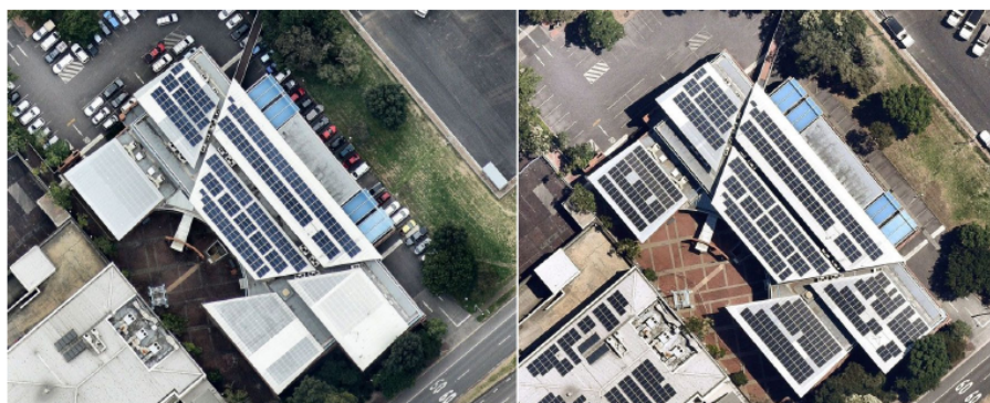
Figure 2: Council Administration Building PV solar array expansion completed in 2022.
