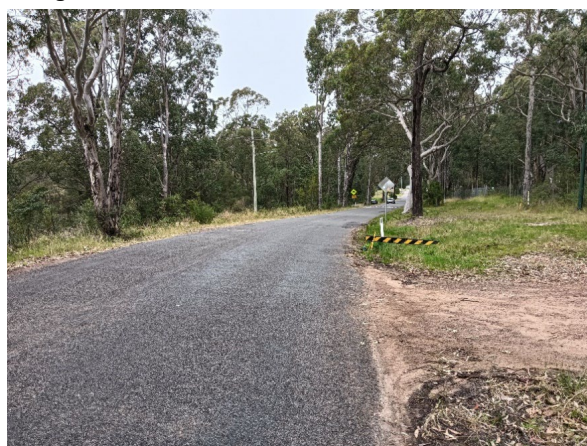
Figure 4 – View of southern section of Mustons Road
