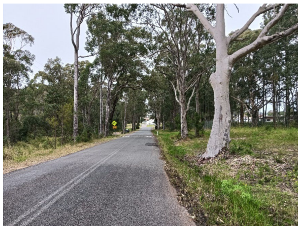
Figure 3 – View of southern section of Mustons Road
