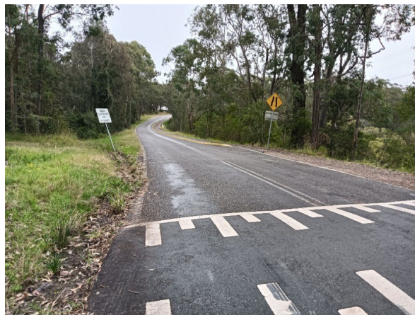
Figure 5 – View of central section of Mustons Road
