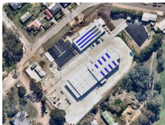
FIGURE 16: RAYMOND TERRACE WORKS DEPOT
