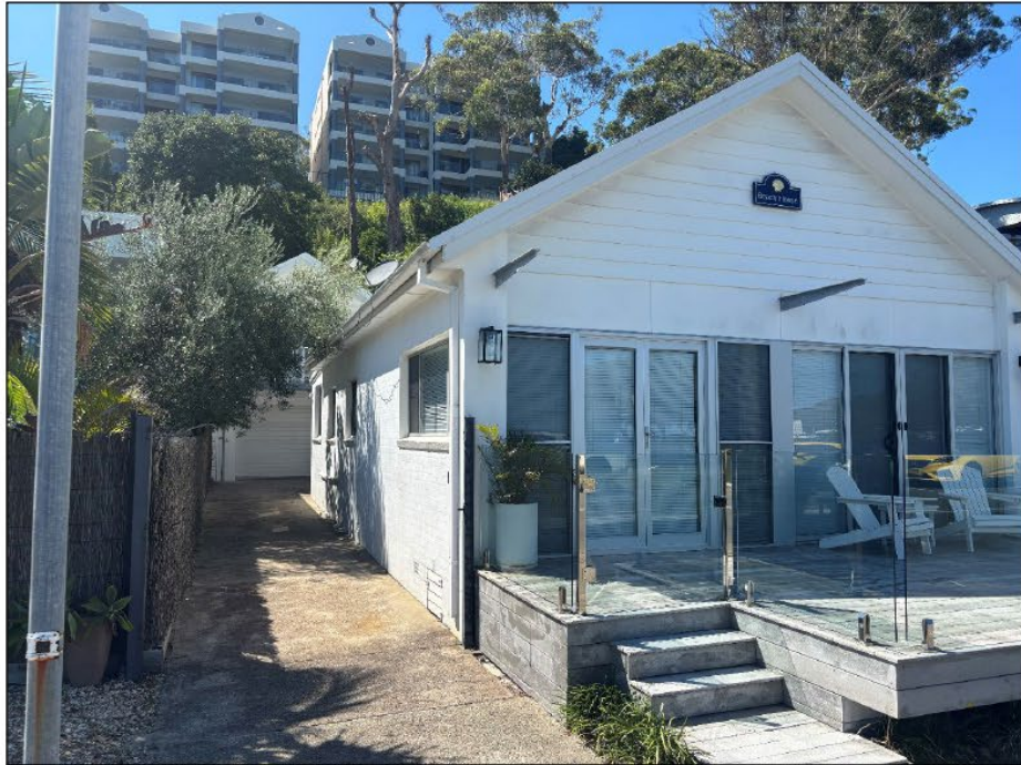
Photograph 2: View along north-east boundary.
