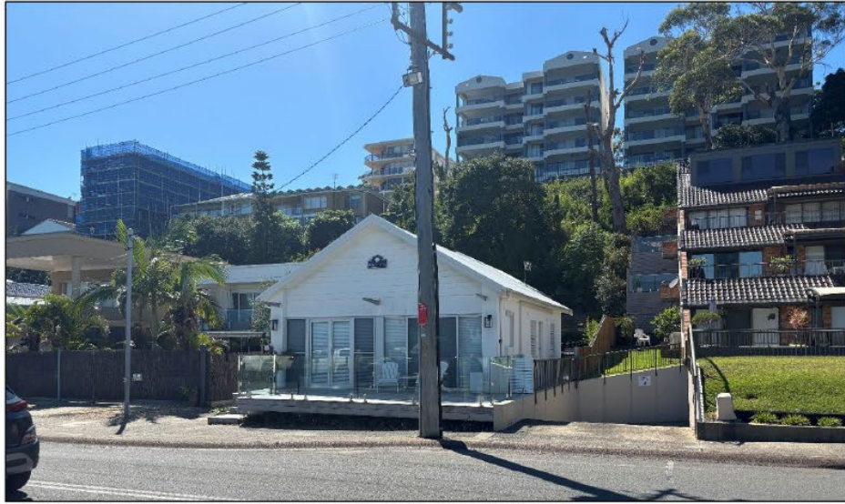
Photograph 1: View of existing dwelling from Victoria Parade.
