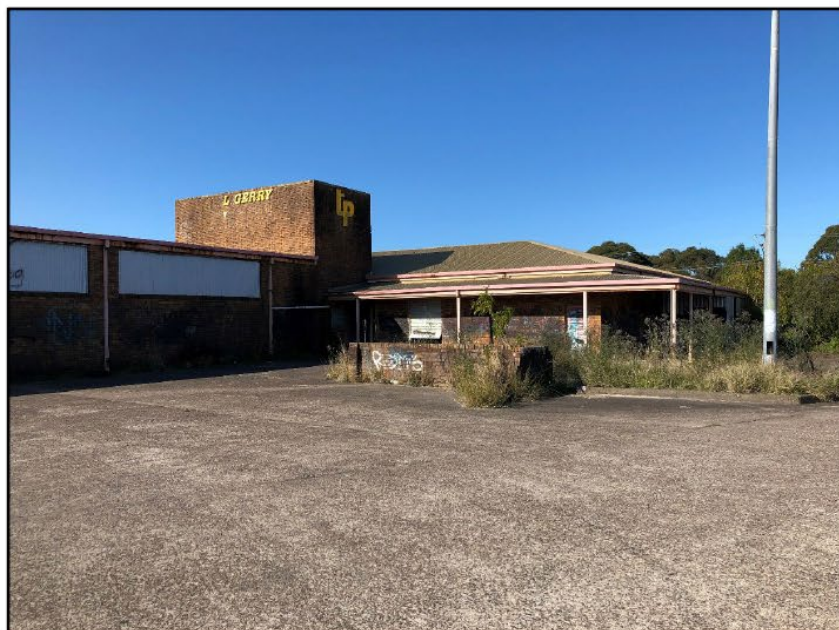
Image 1: Existing building (now removed under demolition order)
