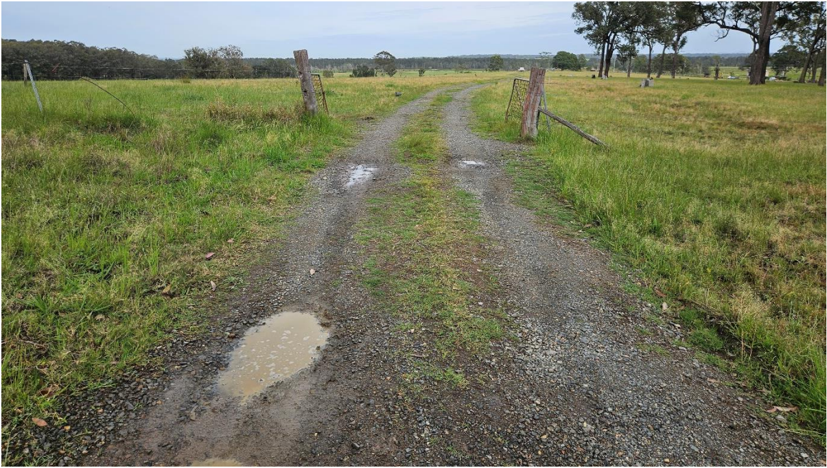
Plate 13. Waterlogged vehicle track. (Source: Heritage Now 2024)
