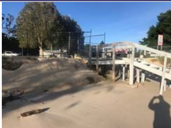
Before and after photos showing placement of sand to address undermining of stairs at Nelson Bay Beach. The sand was sourced via dredging of Little Bay boat ramp, where accreted sand was impacting the use of the boat ramp.
