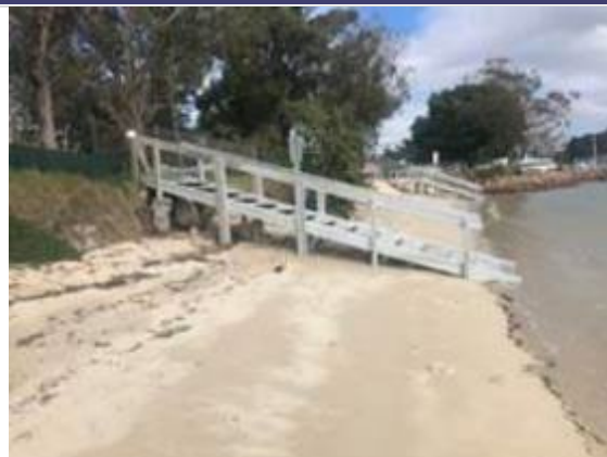
Before and after photos showing placement of sand to address undermining of stairs at Nelson Bay Beach. The sand was sourced via dredging of Little Bay boat ramp, where accreted sand was impacting the use of the boat ramp.
