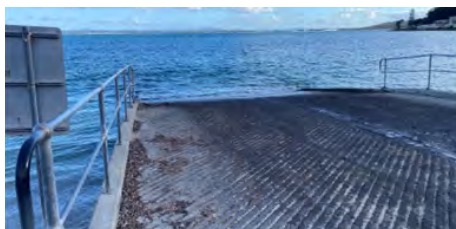
18 Boat Ramps (31 lanes)
