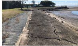
Repair existing seawalls
