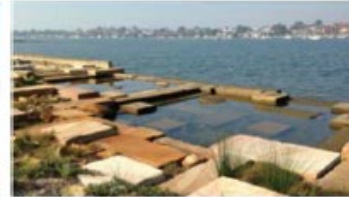
Terrace seawall (with rock pools)
