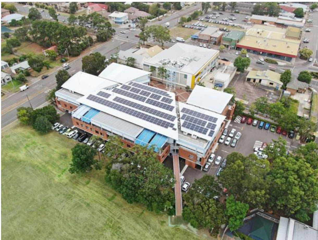
Photo: Solar panels on Council Administration Building
