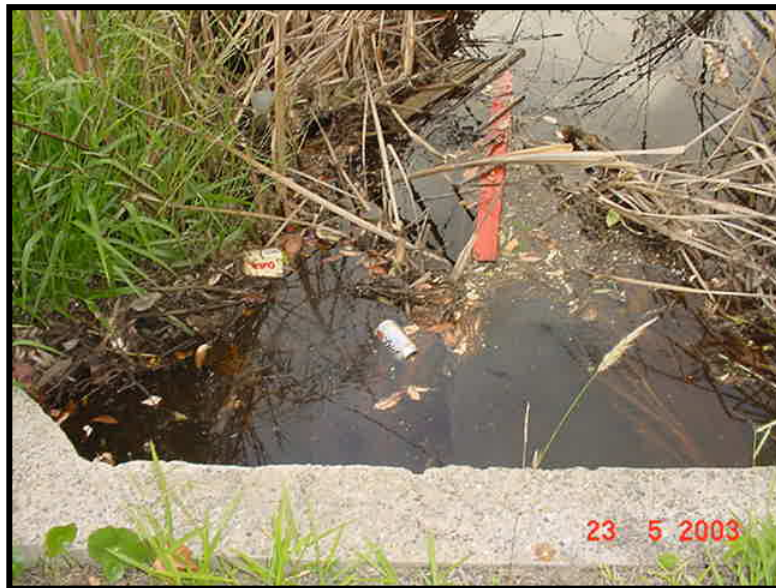
Figure 18: Accumulation of litter in stormwater outlet entering Mambo Wetland.
