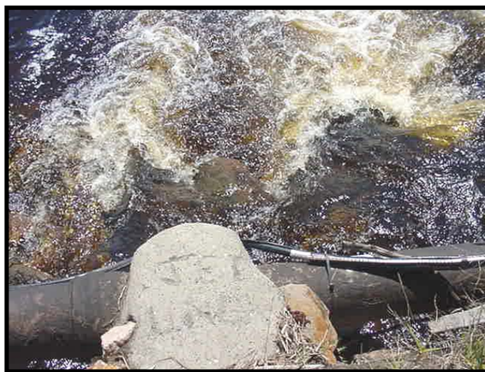
Figure 19: Stormwater outlet at Mambo Creek during high volume flow.
