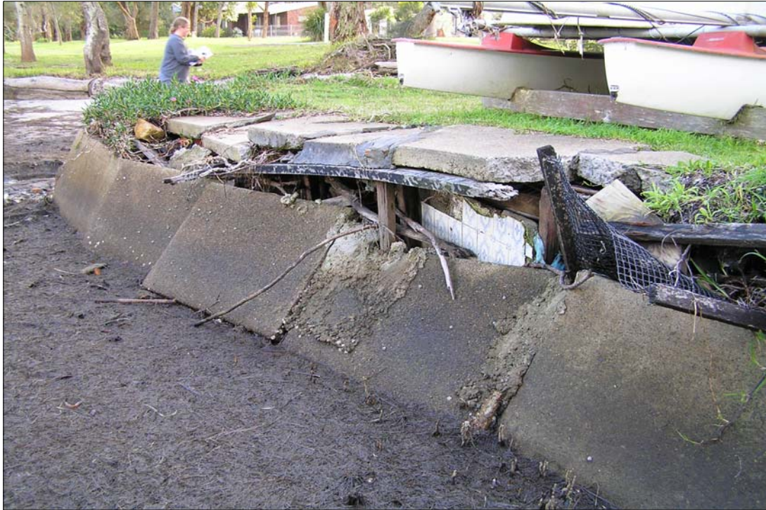
PLATE 7.7 Inappropriate foreshore stabilisation on the lower Tilligerry Creek (Lemon Tree Passage)
