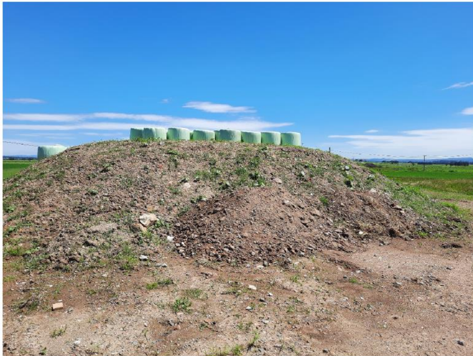
Figure 7: Additional fill to be compacted and levelled over earth mound
