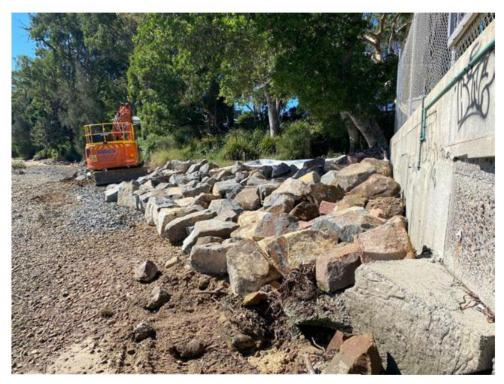
Pictured: Construction of new revetment rock wall at Soldiers Point
