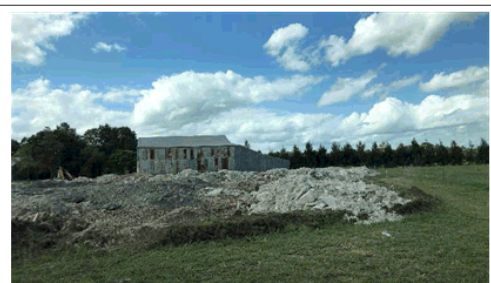
Photo 3: Looking East, approved mound being constructed, proposed site of development and existing metal shed
