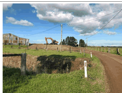
Photo 4: Looking South, approved mound being constructed, proposed site of development
