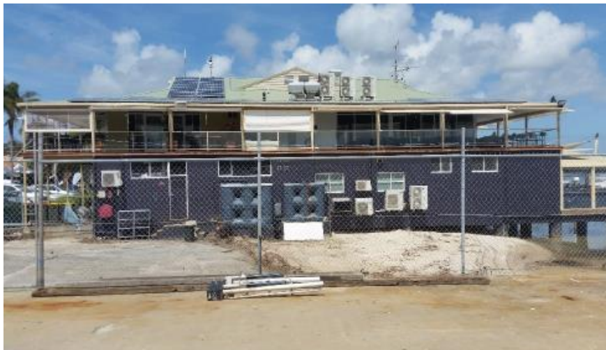
Image 6: Photograph looking south towards the existing club and commercial building with the existing slipway in the foreground.
