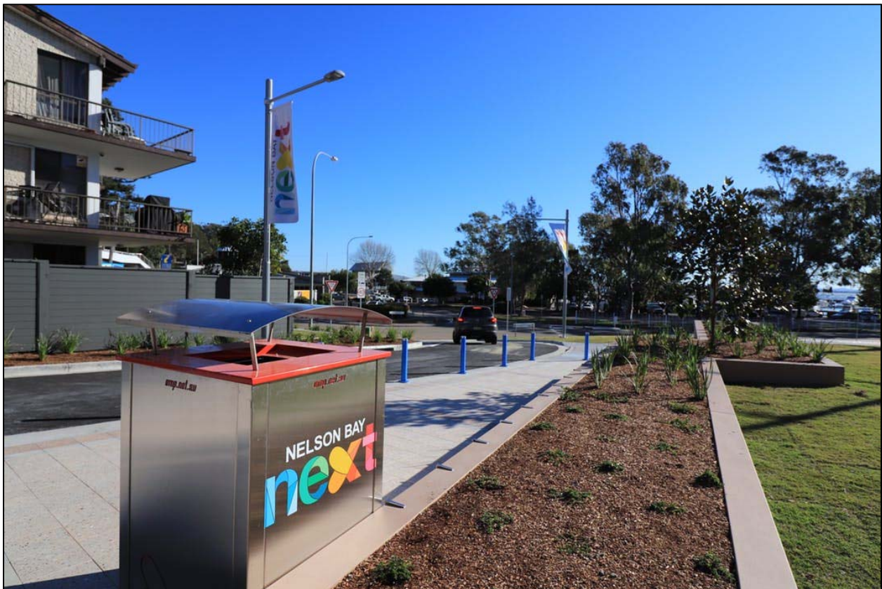
Photo – Yacaaba Street Extension (Source: Port Stephens Council Website)
