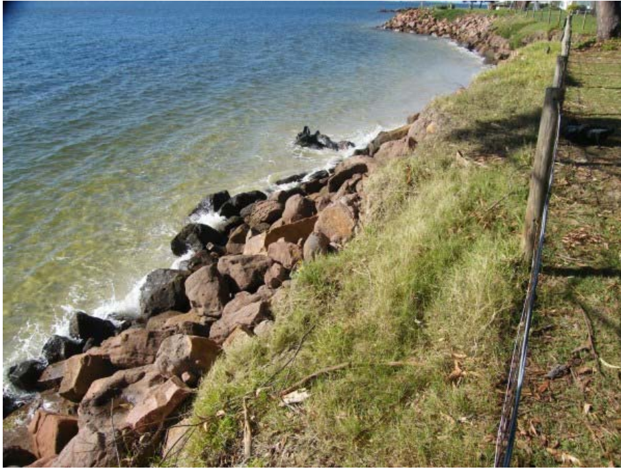
Figure 7 Precinct 3 eastern end Conroy Park. Rock protection has been placed along this section of the foreshore to the western most groyne. Photo Source: D Lord, 8 th May 2015
