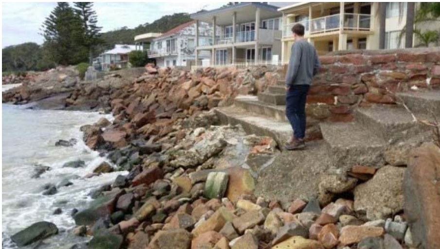
Figure 14 Eastern end of Precinct 5. Sections of the wall have undersized armour, grouted stones and various access stairs and ramps across them. Precinct 5 is the most exposed section of the foreshore and the protection provided is poor for the level of exposure. Photo Source: D Wainwright, 12 th May 2015
