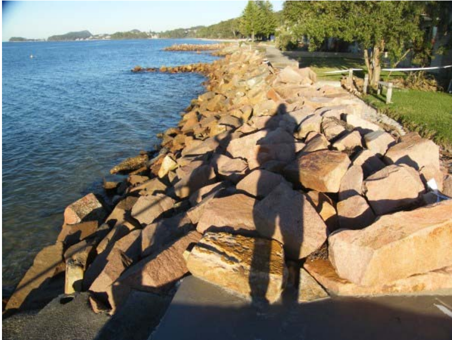
Figure 13 Much of the rock wall along Precinct 5 comprises substantial sized stone at a flatter slope. This is the most exposed section of the study area receiving ocean swells entering the Port during storms. At the time of inspection damage to the wall including loss of armour from the face and crest was observed. Scour holes under slabs and through the wall from overtopping was evident at a number of locations. The alongshore access was closed (SES tapes) along several sections. Photo Source: D Lord, 8 th May 2015
