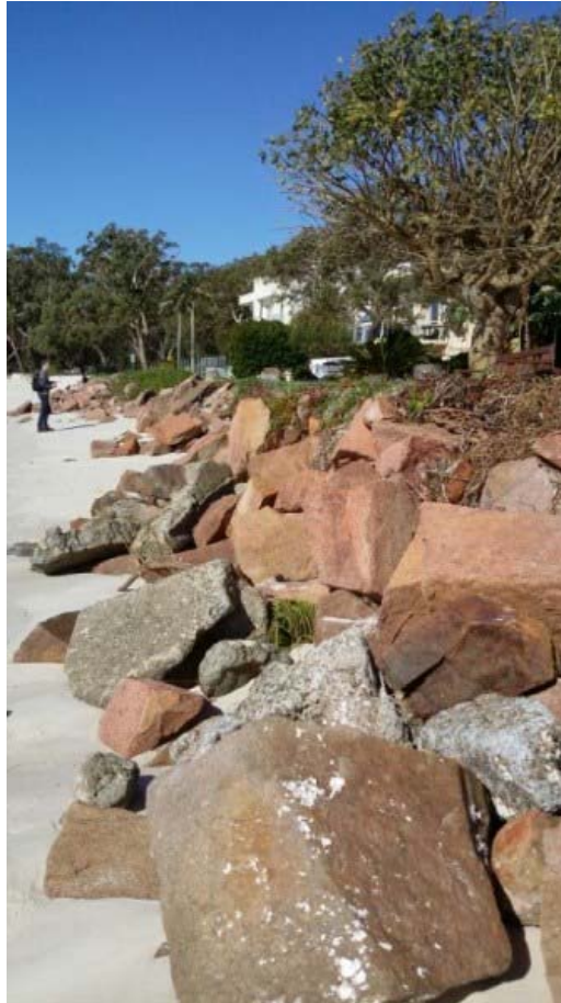
Figure 16 Precinct 6. Some larger rock has been placed along sections of this precinct and a sandy beach remains seaward of this protection work.
