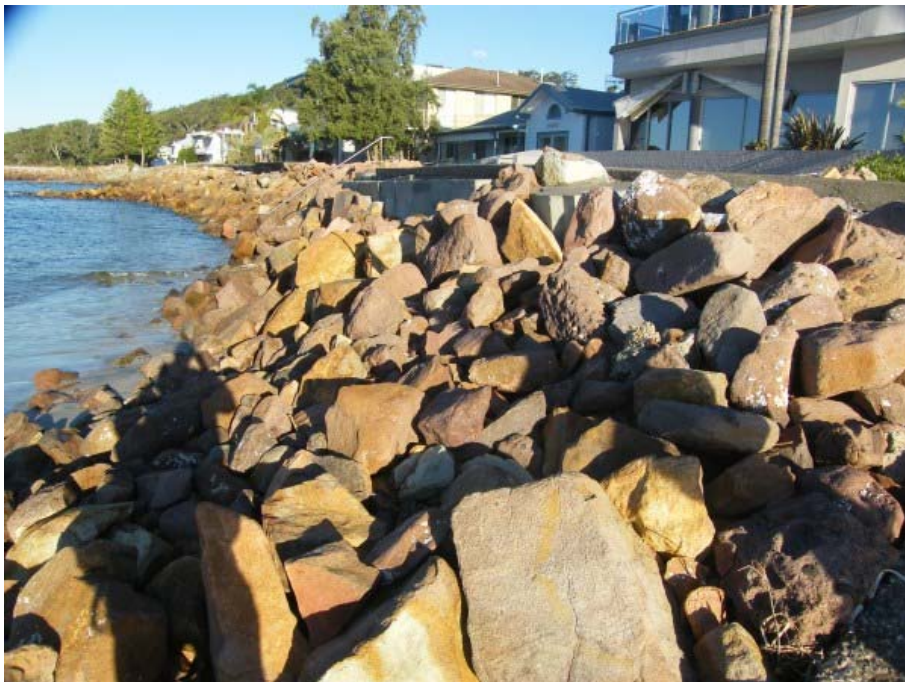
Figure 12 Western end of Precinct 5. A vertical concrete block wall has been constructed in the centre but this precinct is predominantly tipped rock. Little or no sandy beach remains, even at low tide. The public access through Precinct 5 is compromised and wave overtopping during storms is resulting in damage and inundation of property landward of the wall.
