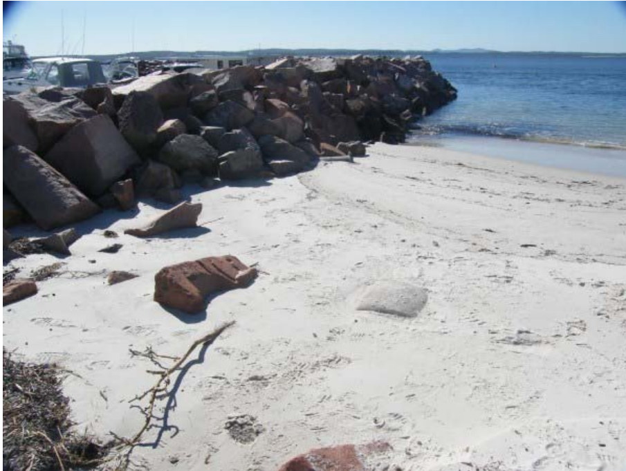
Figure 2 Western end of Precinct 1. Sand accretion against the Anchorage marina wall is burying stormwater outlets. Photo Source: D Lord, 8 th May 2015
