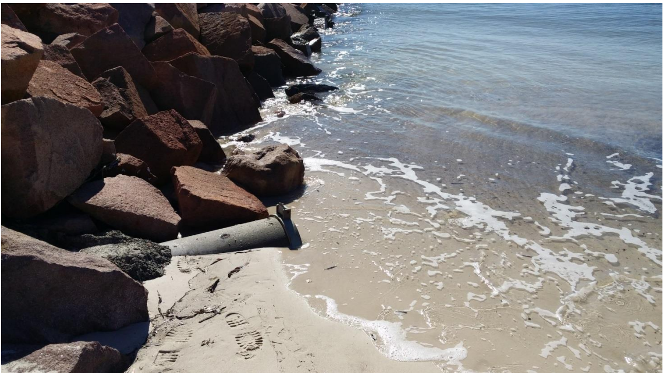
Photo 5 - Outfall 5, partially blocked with flap valve removed.
