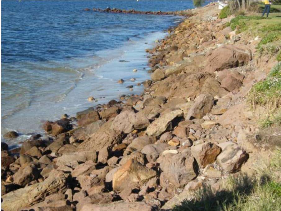
Figure 10 Precinct 4 looking east along the revetment face from the western groyne to the next groyne east. Rock armour sizes along this section are variable with significant slumping and loss of armour near the crest, exposing the erodible bank behind. The accreted sand fillet is visible in the lower left hand corner of the photo
