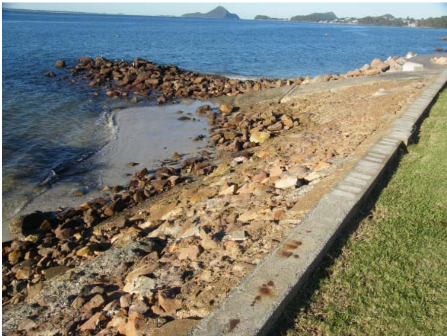
Figure 11 Eastern end of Precinct 4. A boat ramp is located west of the groyne. Rock armour has been grouted to form a smooth wall. The rock groyne has slumped and is too short and low to anchor the beach or provide significant protection. A concrete apron can be seen beyond the groyne in Precinct 5. Photo Source: D Lord, 8 th May 2015
