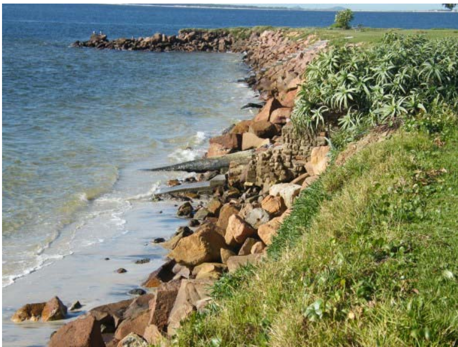
Figure 8 Precinct 3 looking east to the western groyne. Various access stairs of differing design cross the revetment. The wall is generally steep, with some slumping and loss of armour near the crest, exposing the erodible bank behind. Armour stone size is variable. The western groyne and Port Stephens entrance are at the top of the photo. Photo Source: D Lord, 8 th May 2015
