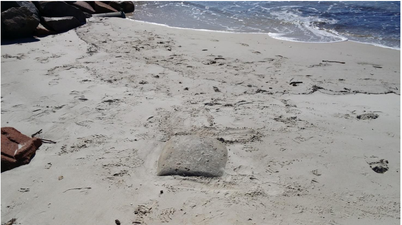
Photo 4 - Outfall 4, completely blocked.
