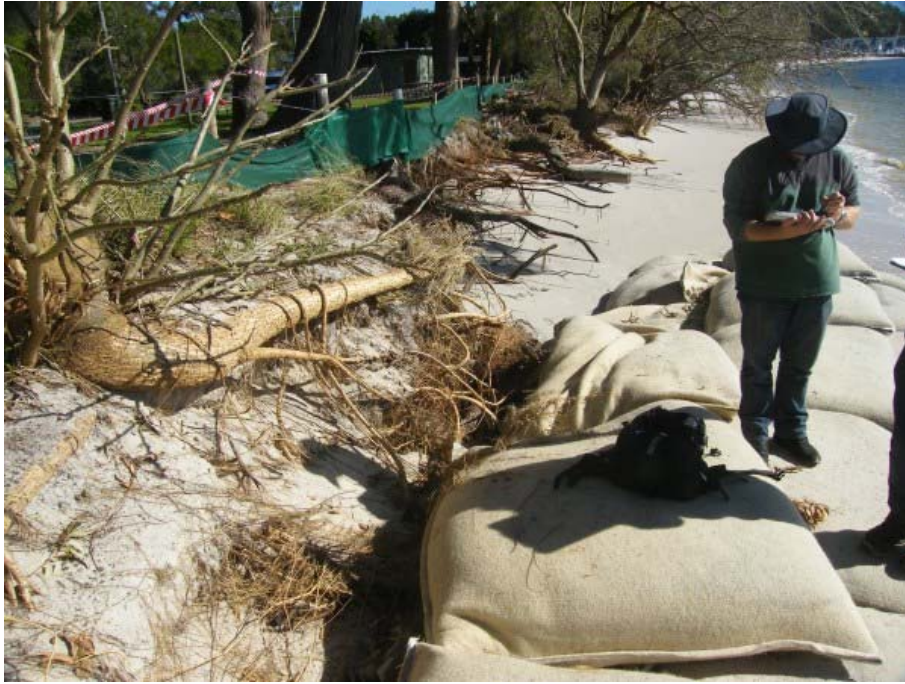
Figure 6 Precinct 2 eastern end. Geotextile containers have been employed for emergency beach protection along the eastern end of Conroy Park. Increased erosion west of the end of the protection is evident. Additional containers have been placed to extend the wall since this photo. There is little sandy beach width remaining at this location and no beach at mid to high tides. Access to the beach from the park has been affected.
