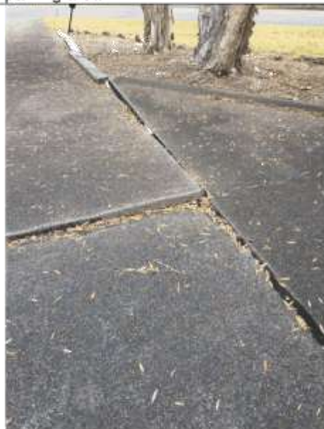
Movement in the car parking slab area was noted. Draft conditions included which require the rectification of the slab movement prior to the issue of an Occupation Certificate.
