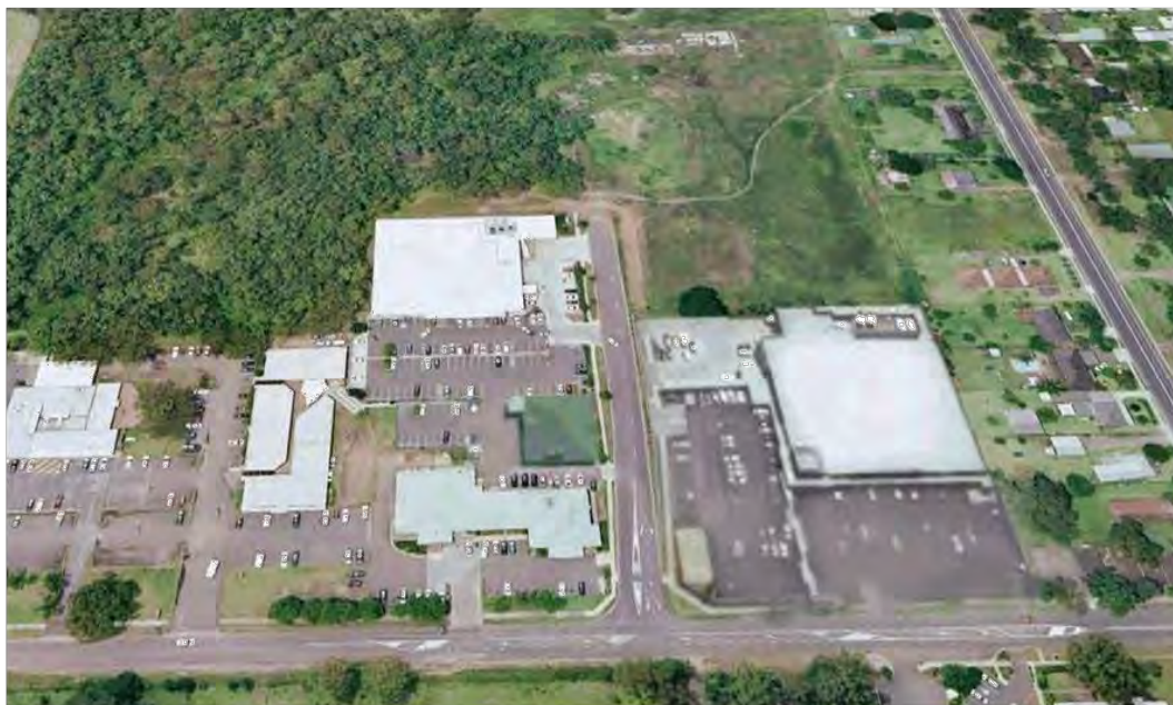
Figure 15: Existing Conditions (Looking North)
