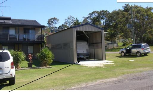
The Location of the shed encroaches building line front setback by 2.65m, side setback and height are non-compliant with the Port Stephens DCP 2013.
