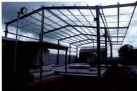
Photo 2 – Close-up view of the partially constructed shed.
