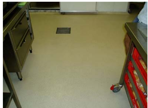
Picture 5: Floor waste
