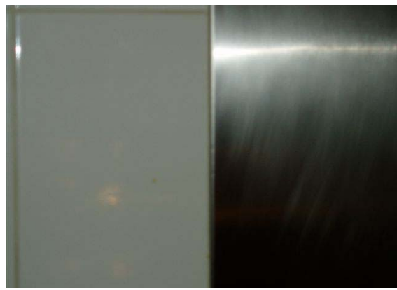
Picture 13: Stainless steel splashback sealed to a tiled wall surface.
