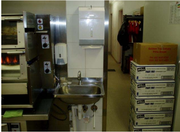
Picture 10 & 11: Hands free operated hand wash basin with paper towel and liquid soap dispenser.
