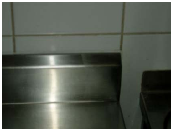
Picture 12: Sealing bench tops to wall.
