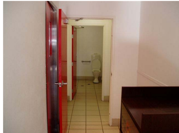
Picture 16: Toilets separated by air lock with self-closing doors
