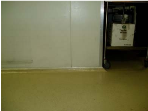
Picture 6: Epoxy coving on a coolroom floor
