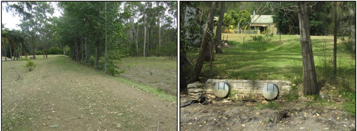
These current levees will need on-going maintenance and checks to ensure they continue to function as designed. It is understood that there have been some drainage issues at the Kirrang Drive levee and Council is in the process of rectifying this. Regular maintenance of the existing levees and associated drainage infrastructure should be included as a recommendation in the final adopted FRMP.
