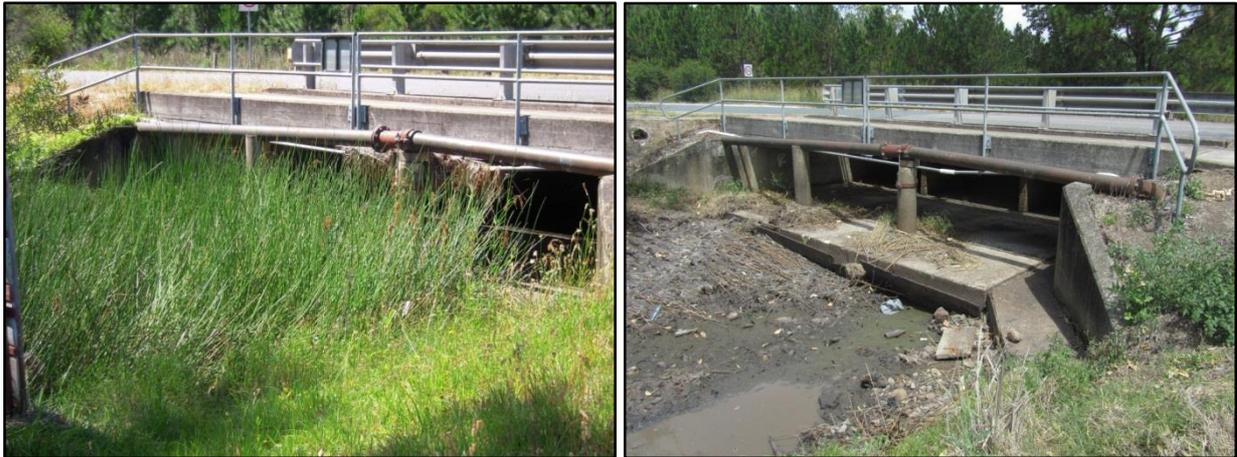
**Photograph 15: a) Vegetation Upstream Of Kirrang Drive Culverts (still to be cleared as of
